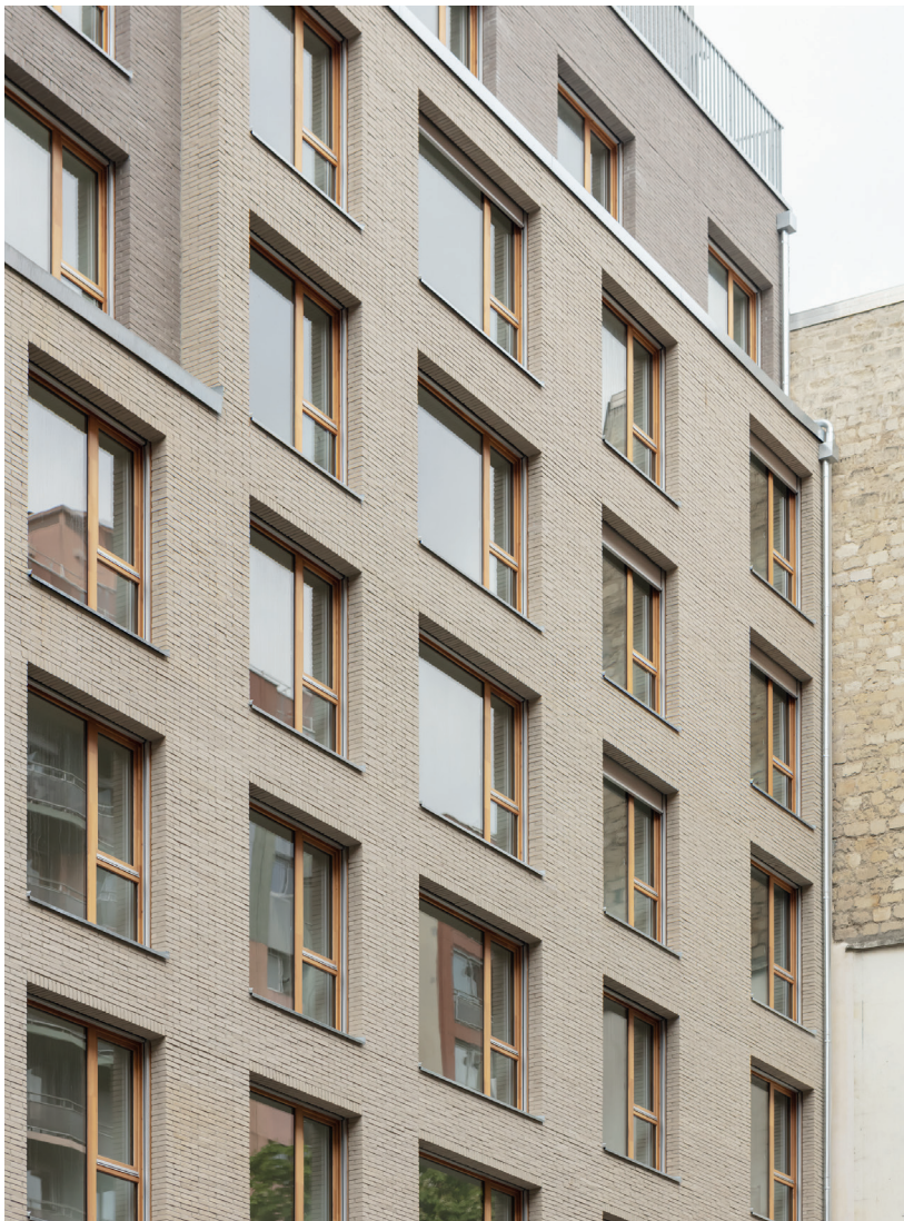
Overall view of main façade on rue Petit and the brickwork on rue Petit as well as the solid wood window frames.
